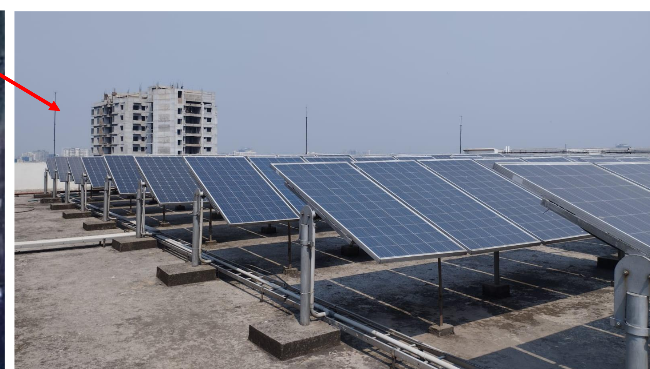
75 kW AC Rooftop PV System installed on the rooftop of ECE Building of BUET
